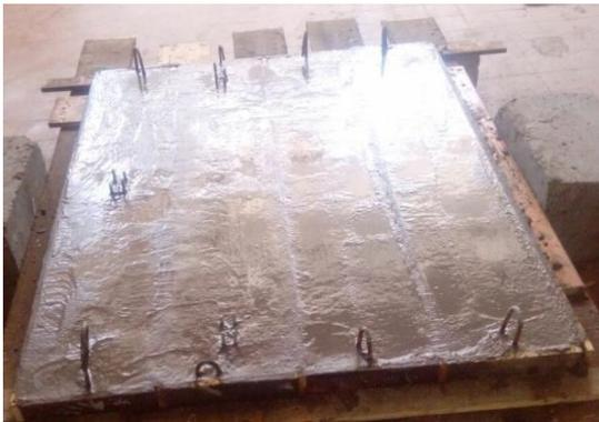
b- Wooden form and reinforcement of concrete slab
